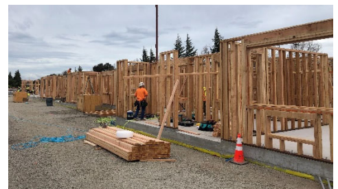
Wood framing going up at the site!
